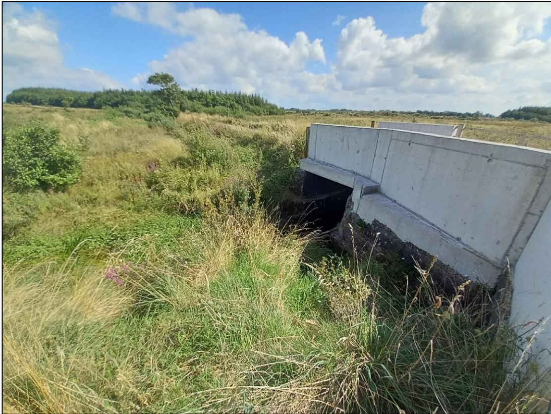
Plate 4-45 Concrete box culvert over the Levally Stream
